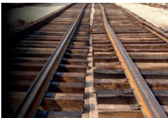
Figure 19.15 (a) – Sleepers on railway line
