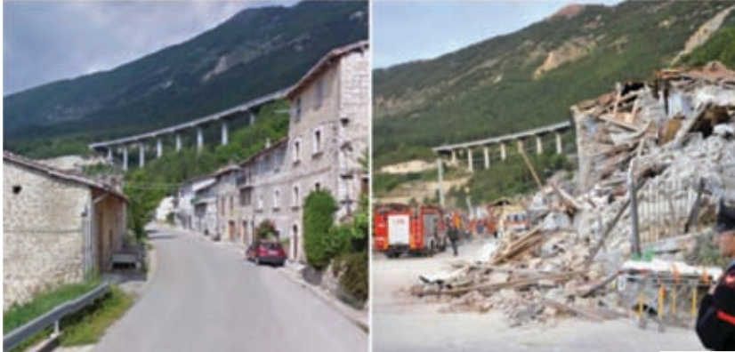
Figure 18.6 – Photographs of the same area before and after the Earthquake
