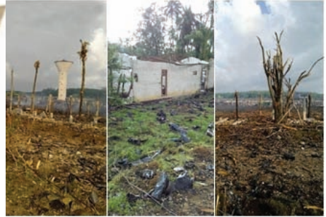
Destruction caused by the explosion of armory in Salawa, Kosgama
