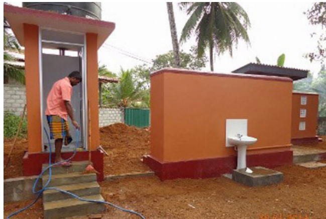
Figure 1.8 - Providing adequate sanitary facilities
