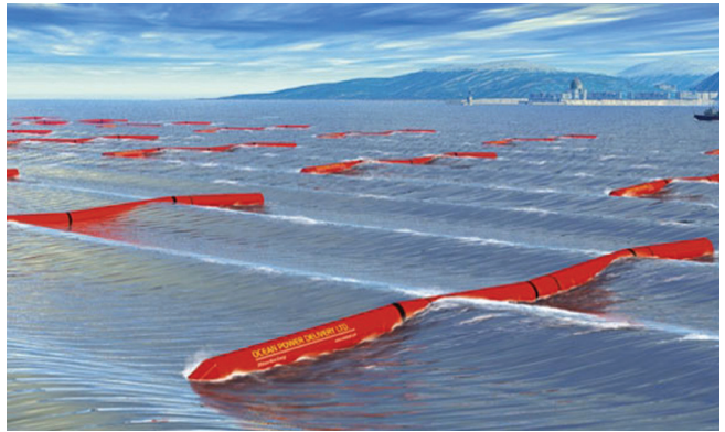
Fig. 4.19 ▲ A power station operated by sea waves
