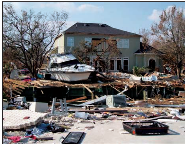
Fig 5.17: A destroyed area
