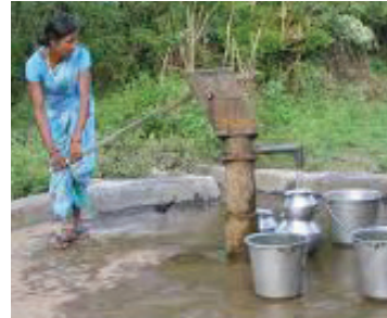
Installing tube wells
